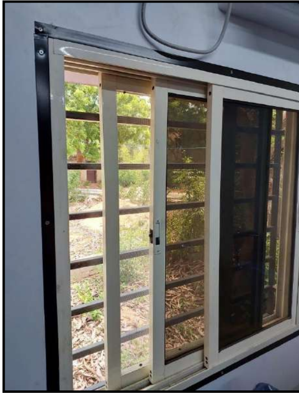
(THREE LAYERS WINDOW DESIGN)
