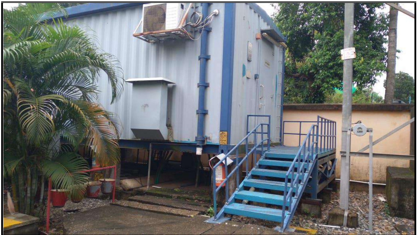
(MAIN PORTACABIN OUTSIDE VIEW)
