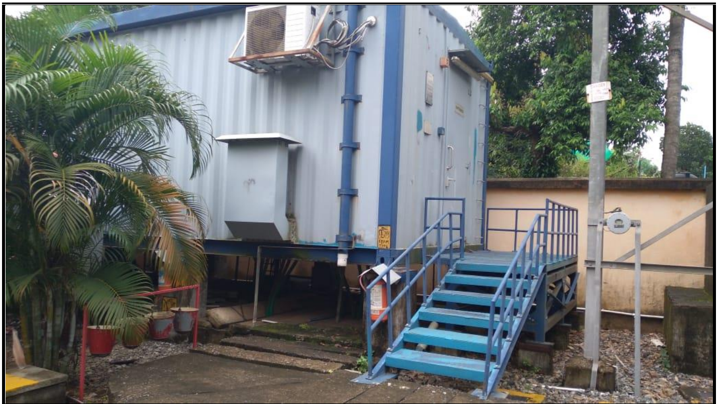
(MAIN PORTACABIN OUTSIDE VIEW)
