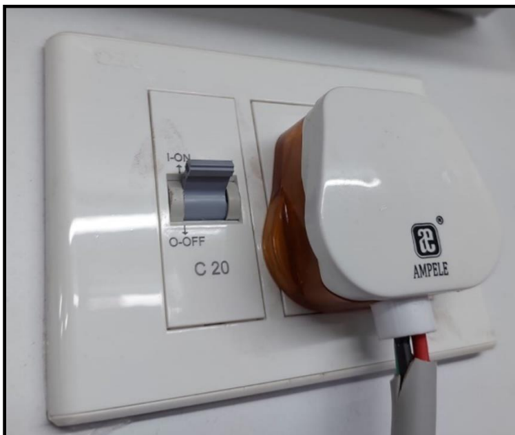
MCB, 3PH ELCB & PLUG POINTS , ELECTRICAL APPLIANCES OF PORTACABIN
